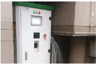
Power Grid Corporation of India Ltd (PGCIL) Location - Jammu-180004 (J&K) Capacity - 15kW GBT DC fast charger
